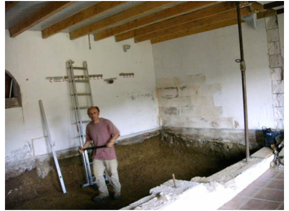
Michel digging, the wall now completely torn down.
