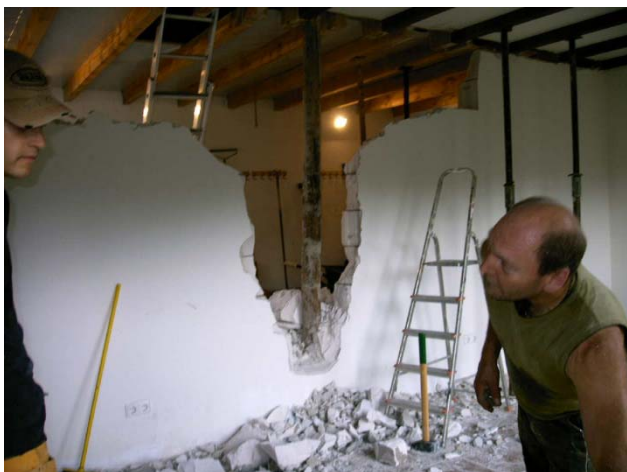
Jochem & Ralph before the wall, half broken down
